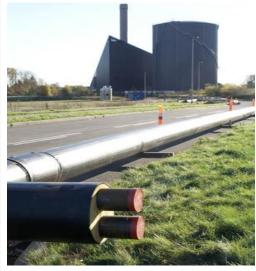
Twin pipe DH pipe system © Logstor Higher performance systems exist that reduce the heat distribution losses relative to the use of single pipe systems, *e.g. twin pipes*
