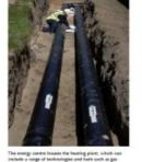
boles, biornes boles and contoined heat and priver (CHF). Hot water from the energy centre is pumped through the pipe restruct to the individual buildings, in each divelling, heat is conveyed via the hydraulic interface with to the central beating statutors and to the hot water tags of gave 21.
