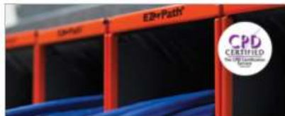
FIRE STOPPING: BREAKING THE CYCLE OF NON-COMPLIANCE
