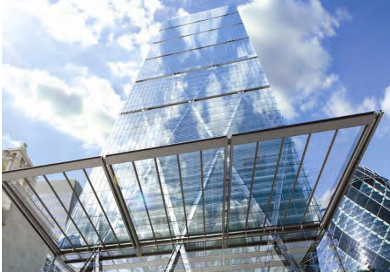
Figure 1.5: No. 122 Leadenhall Street
