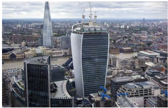
Figure 1.2: No. 20 Fenchurch (Alden 2013)
