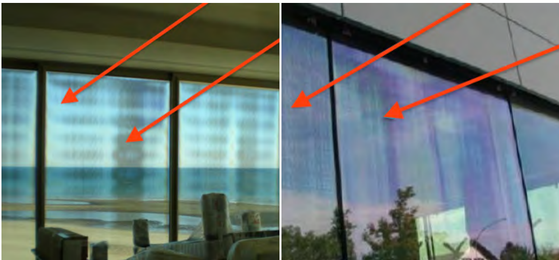
Figure 3.3.10: Anisotropy caused by quench (Narrow) and furnace (Wide) (Vehmas 2014)
