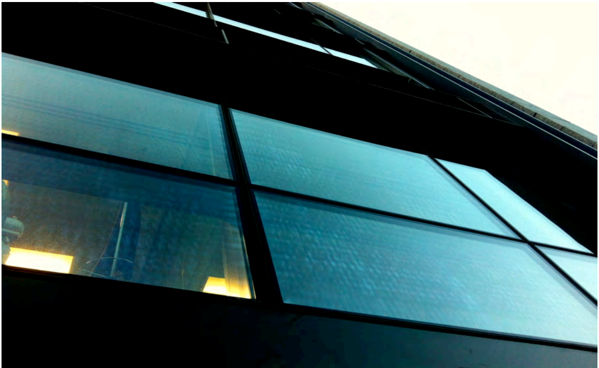
Figure 2.1: Anisotropy or leopard spots in heat-treated glass
