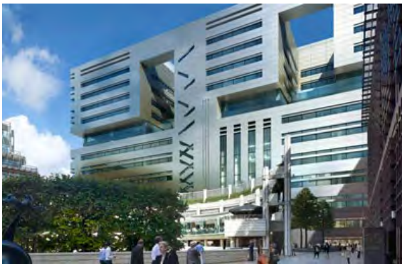
Figure 1.1: No. 5 Broadgate (Kollewe 2011)
