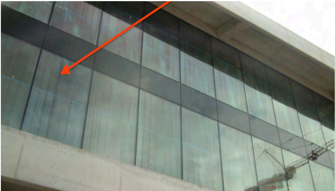
Figure 3.3.9: Anisotropy caused by convection issue in furnace (Vehmas 2014)
