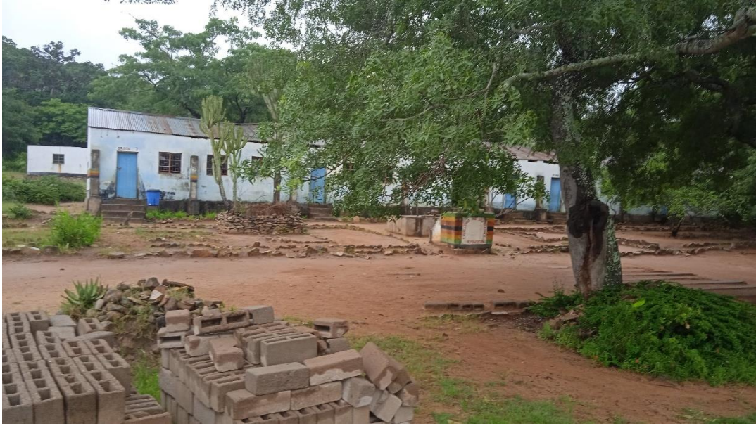
Figure 1: School building at Gorondondo Primary school
