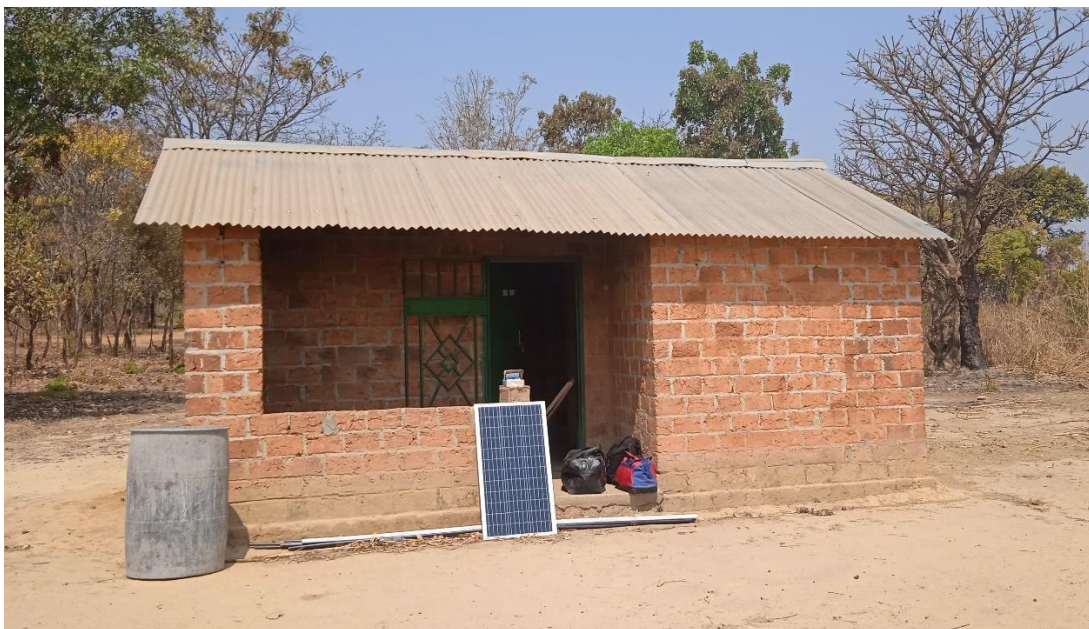
Figure 17 :Installing the solar panel on a residential building in Zambia
