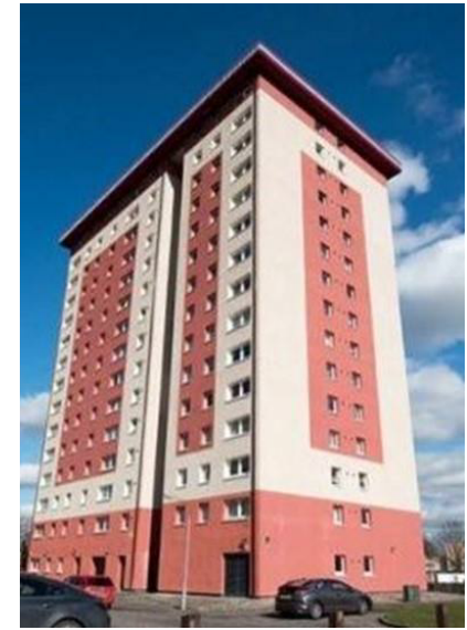
150 electric hot water tanks replaced by Heat Battery
