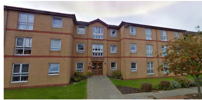
Small district heating with Heat Battery
