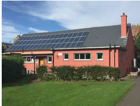
Village Hall with PV, 2x heat pumps and PV
