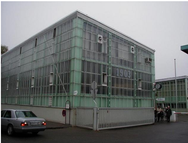
Figure 3.1, The Steiff Factory (Blasco, 2012)
