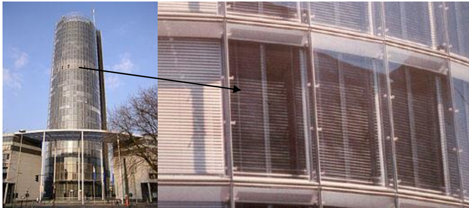
Figure 3.2, RWE Building (BESTFACADE, 2008) Figure 3.3, RWE, closer detail (BESTFACADE, 2008)
