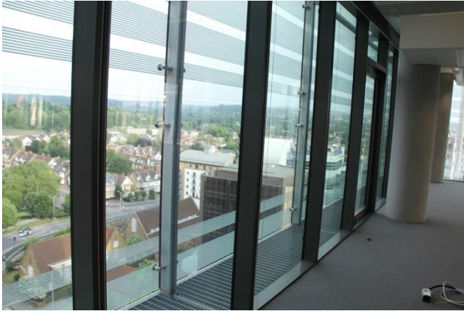
Figure 6.2 Unitised CW (viewed internally)
