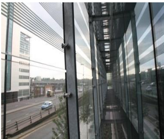
Figure 3.14 Multi storey cavity
