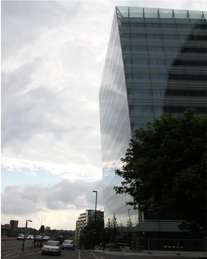
Figure 6.19 South East corner adjacent main arterial motorway
