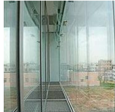
Figure 3.13 Corridor Cavity (BESTFACADE 2008)
