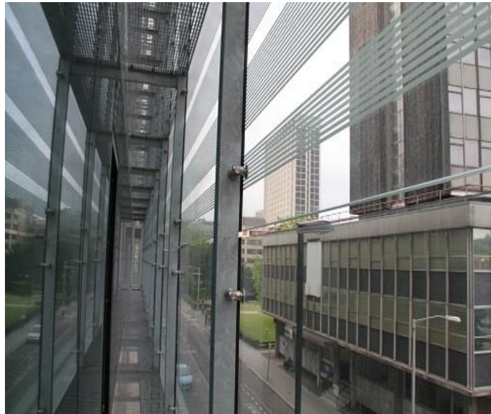
Figure 6.3 30mm gap on external skin
