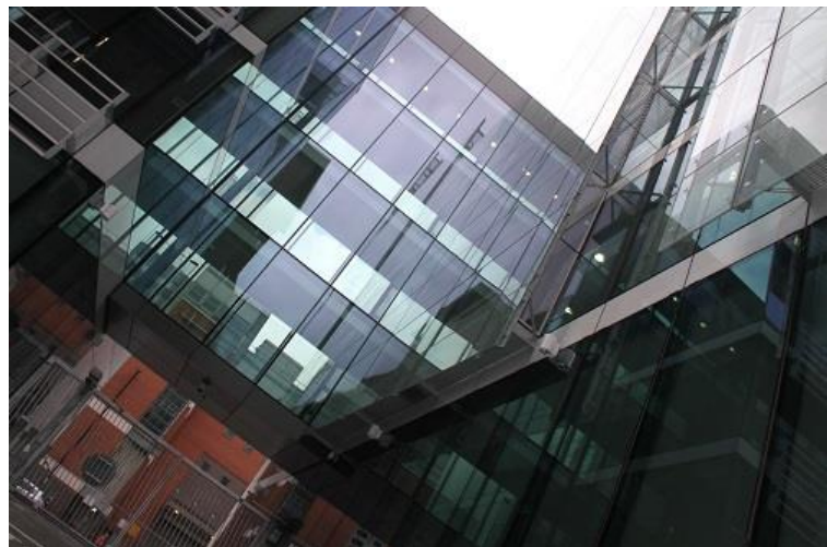
Figure 6.20 Link Bridge (lowest L_{Aeq} readings taken behind the bridge near the red brick building)
