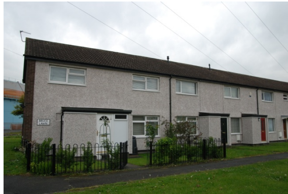
After (external insulation)
