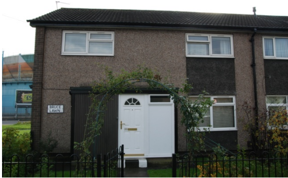
Before (external insulation)
