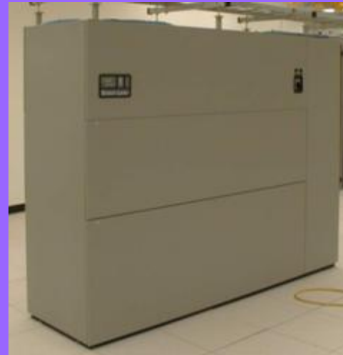
Computer Room Air Conditioner (Circa 1980)
